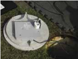
AMR/AMI meter transmitter units (MTU) are often buried underground, exposed to extreme temperatures and difficult to access for replacement. Bobbin-type LiSOCl 2 cells with passivation minimize the need for future battery replacement, which increases ROI.
