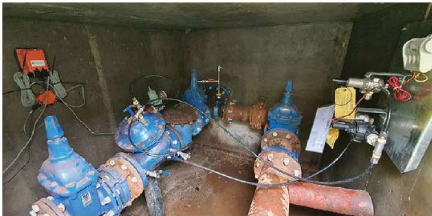
2. Erie County in Pennsylvania uses AI-enabled, battery-powered Wavelet devices to monitor pressure-reducing valves to protect a 100-year-old water system.
