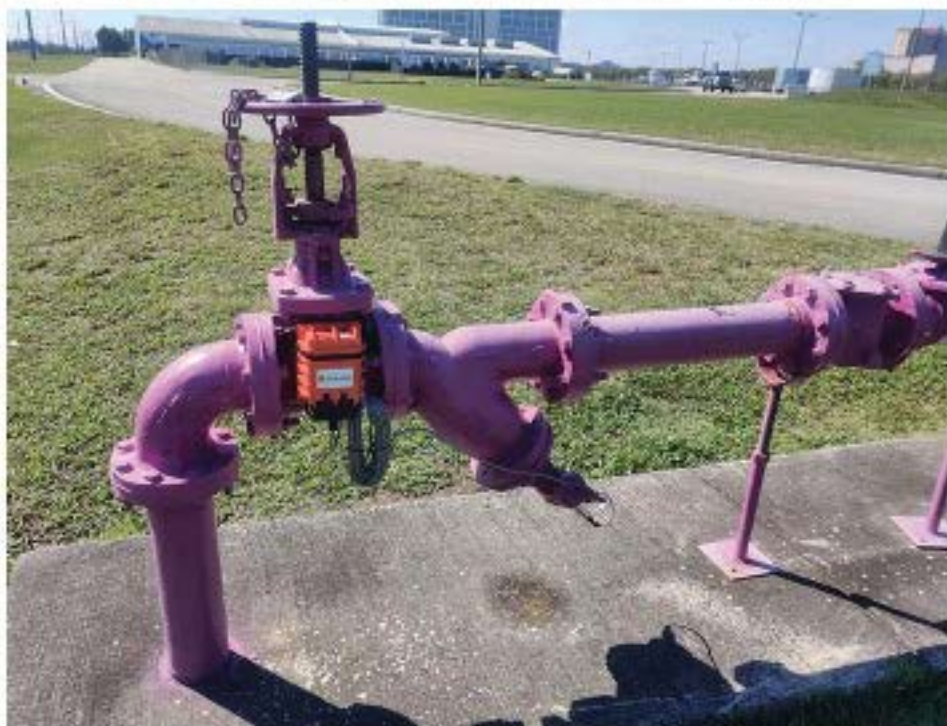
1. Florida's Orange County uses Ayyeka Wavelet devices equipped with Tadiran high-energy \text{LiSOCl}_2 batteries to manage the distribution of reclaimed water to golf courses, resorts, and homes.
